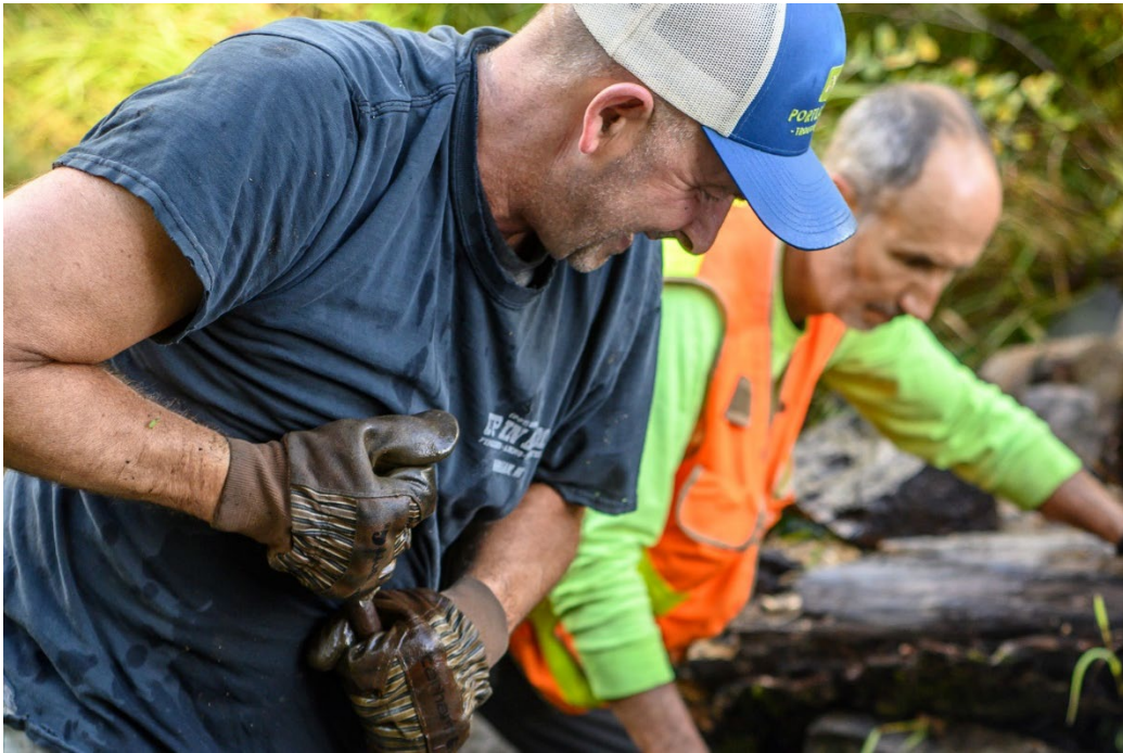
BURGESS BROOK DAM REMOVAL, SEPTEMBER 2022
