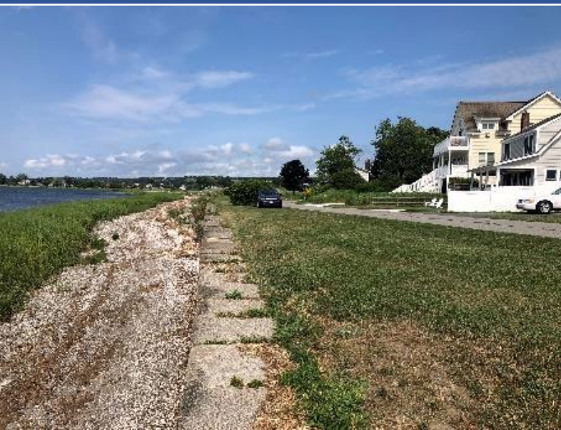
New stormwater filtration area installed by town
