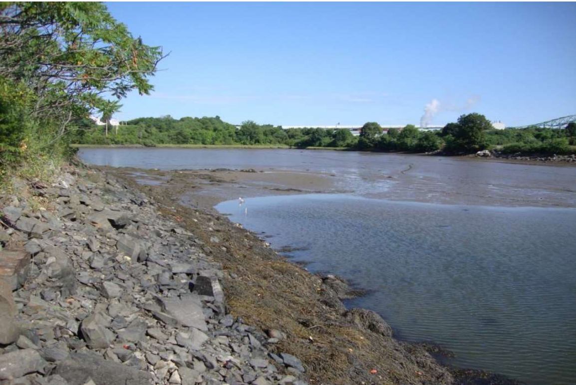
Figure 4.3: Rip-rap along the southern shoreline in Cutts Cove
