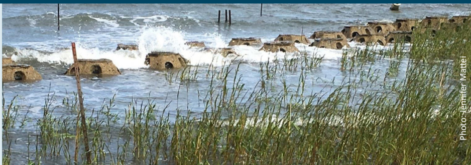
Stratford Point Living Shoreline (reef ball breakwater), Stratford, CT
