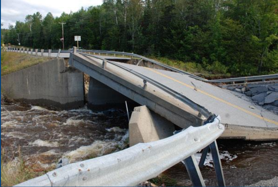
Carrabassett Valley bridge failures, Hurricane Irene, 2011
