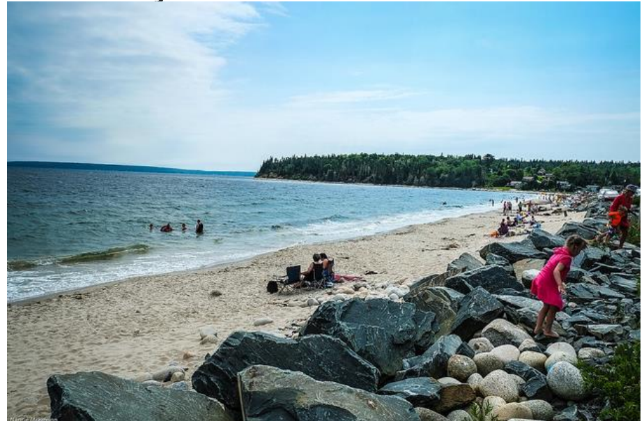
Beach after armour rock installed
