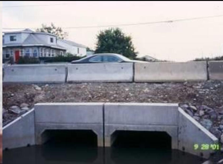
New 48" Twin Box Culvert (adequate flow)
